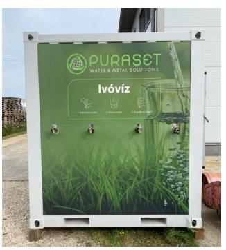
The equipment was installed at two locations in the municipality, where, in addition to supplying the institutions' kitchen drinking water needs, the population could also get drinking water from taps on the side walls of the container. The solution is sustainable and economical temporary water supply type in comparison with other water distribution methods such as plastic bottled water or distribution with water tank cars.
